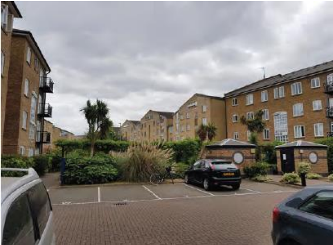
1. View across site from east side of site
