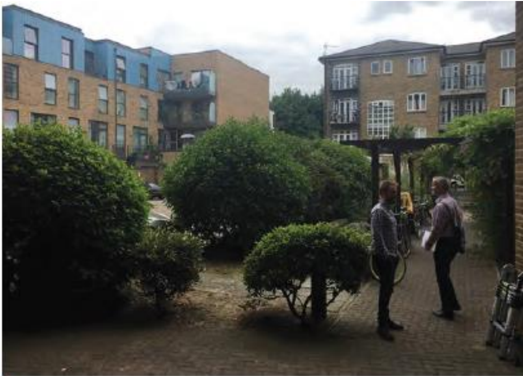
3. View from north west of site looking at Block A
