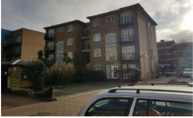
Photograph from site
