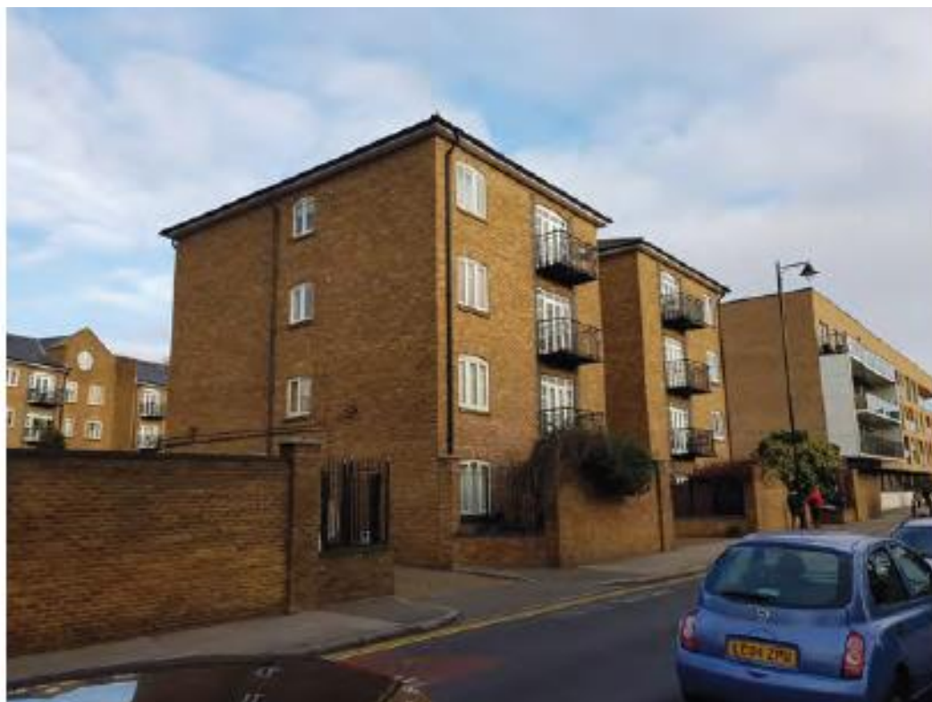
5. View of south facade of Block A (street view)
