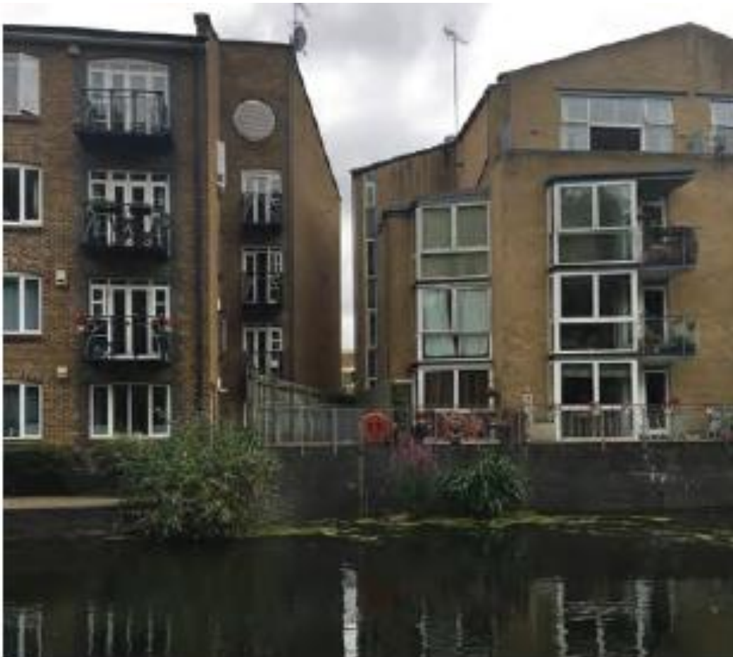
7. View of west side of Block B from canal tow path
