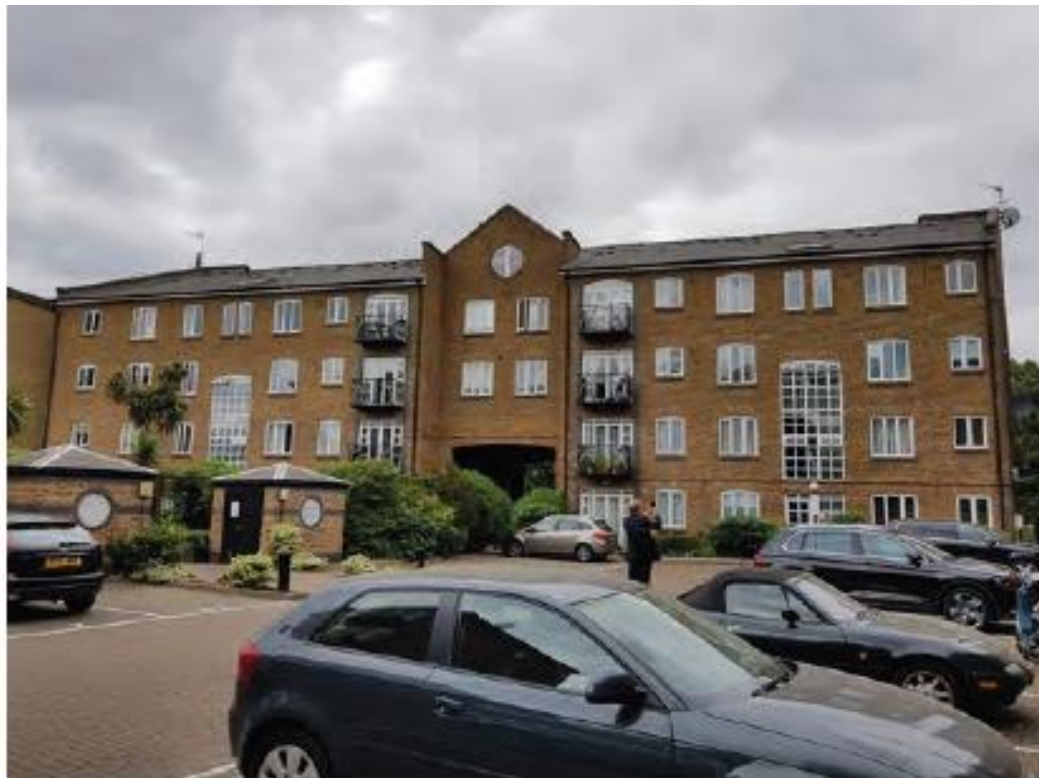
4. View of south facade of Block B
