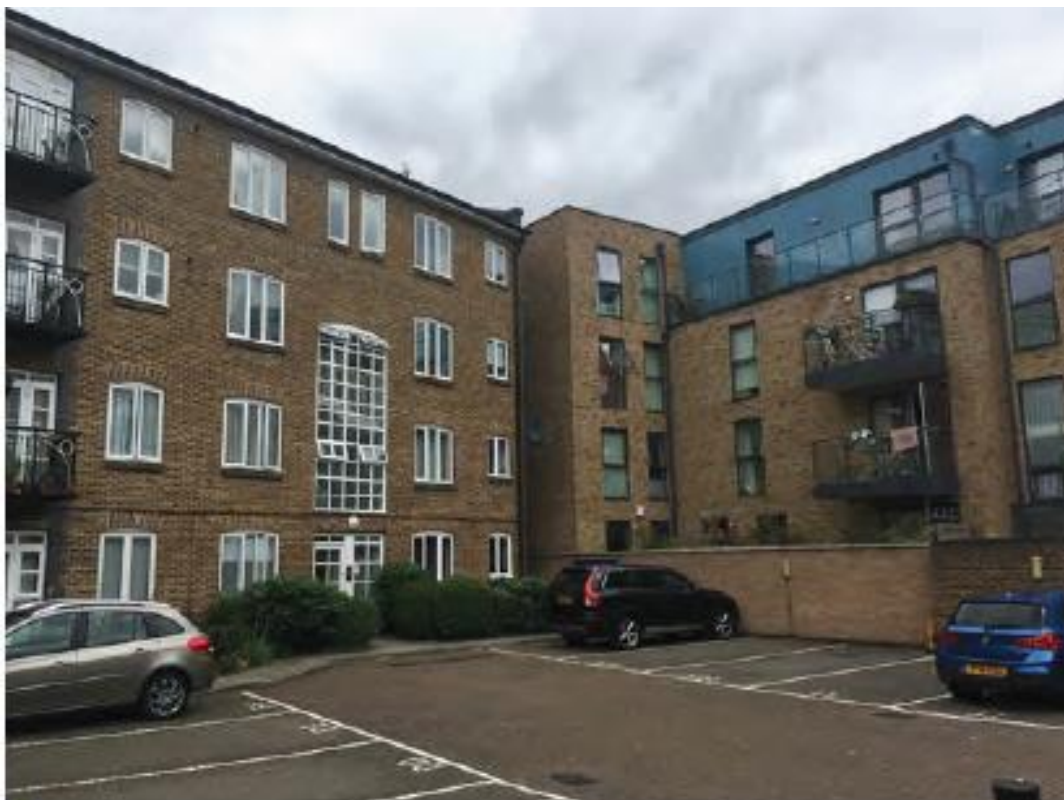
2. View of east side of Block B
