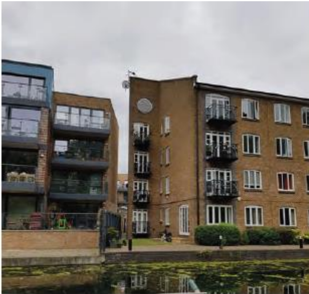
8. View of east side of Block B from canal tow path
