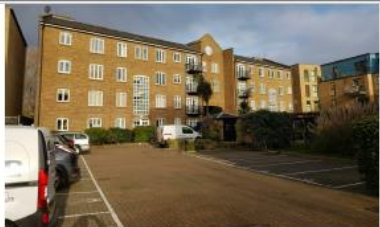
Photograph from site
